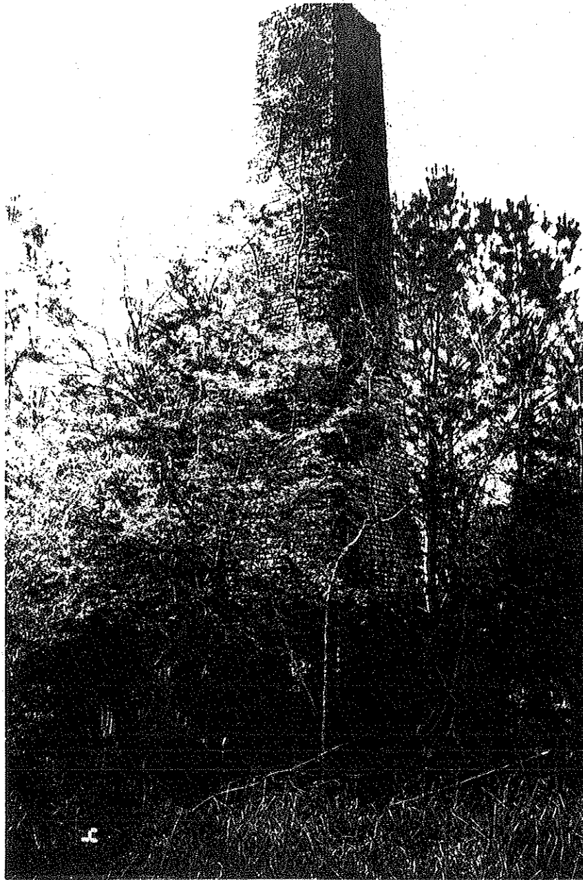
Figure 8. 38CH1075 Standing Boiler Chimney.
